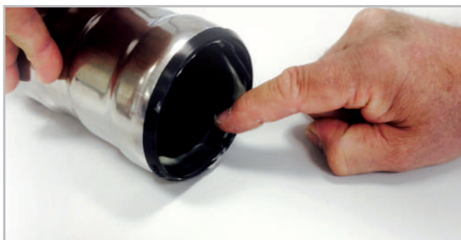
Figure 6 - Internal gasket lubrication
