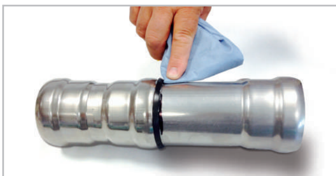
Figure 8 - Cleaning of the grease residual
